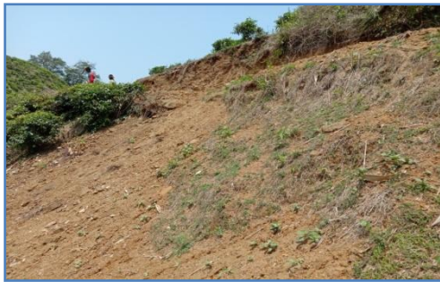
Before installation of JGT at Binnakandy Tea Estate
