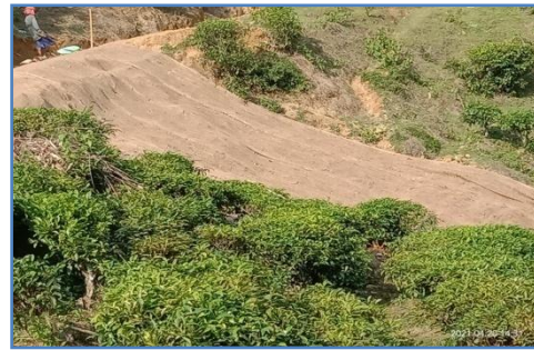
During installation of JGT at Binnakandy Tea Estate
