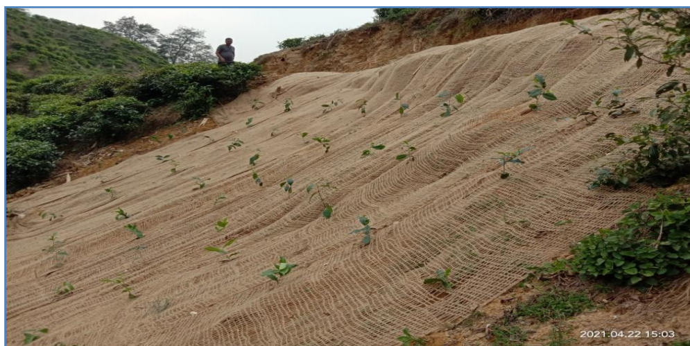
After installation of JGT Material at Binnakandy Tea Estate
