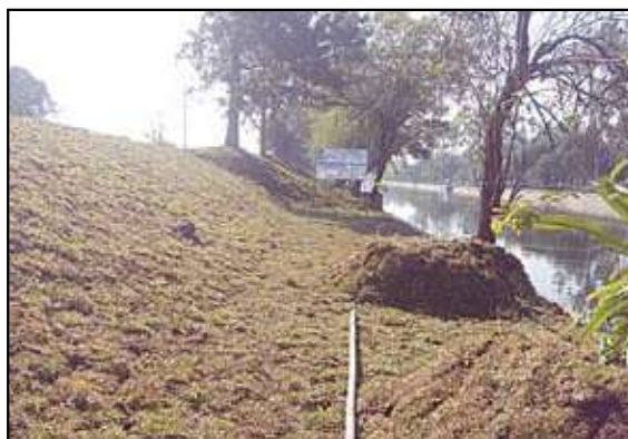
Complete vegetated slope over JGT
