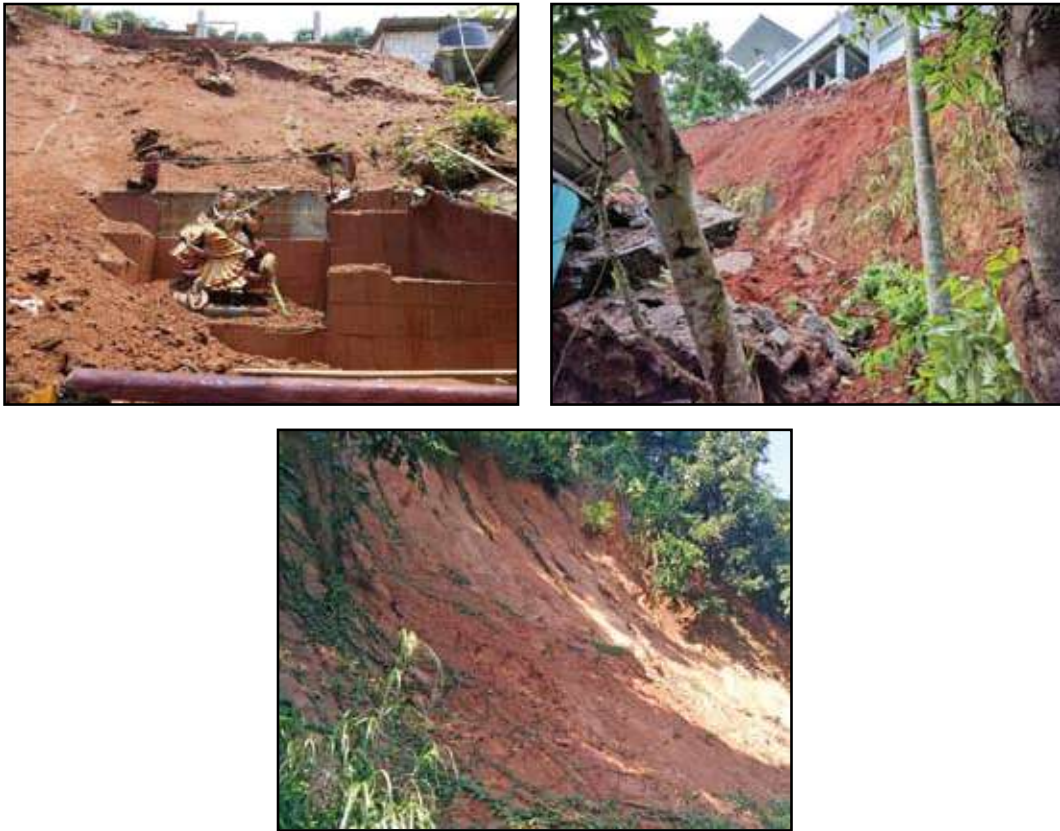
Few of the site snapshots taken during site analysis in Assam
