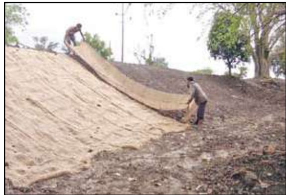
JGT laying on progress
