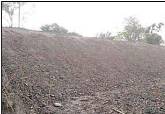
Dressed slope before application
