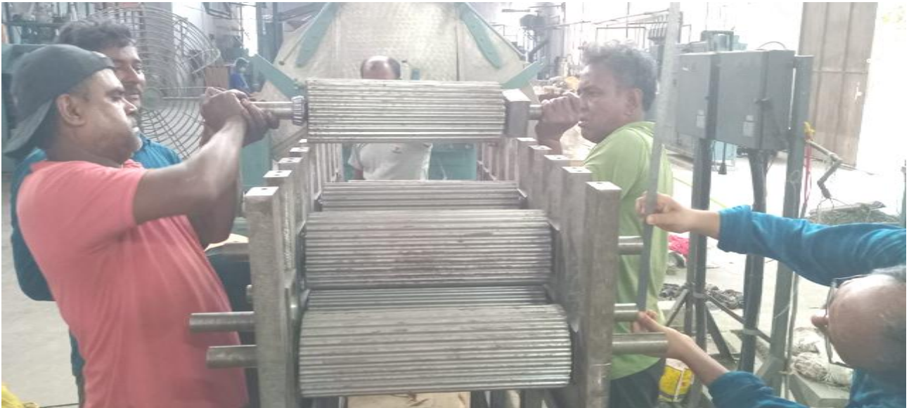
IJIRA's Automatic Fiber Opener (under erection)
