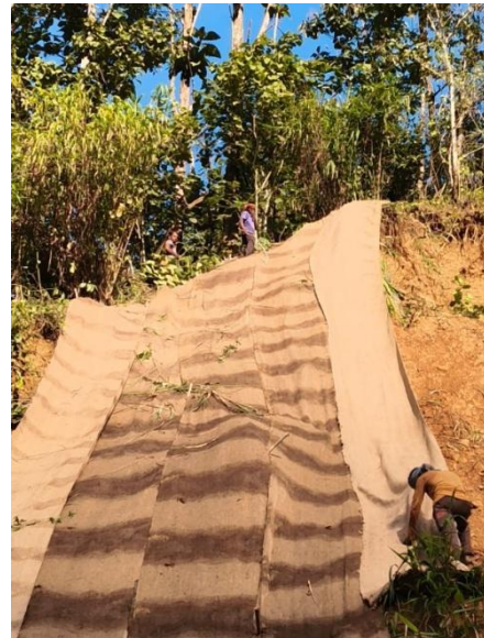
Laying of 1200gsm open weave JGT
