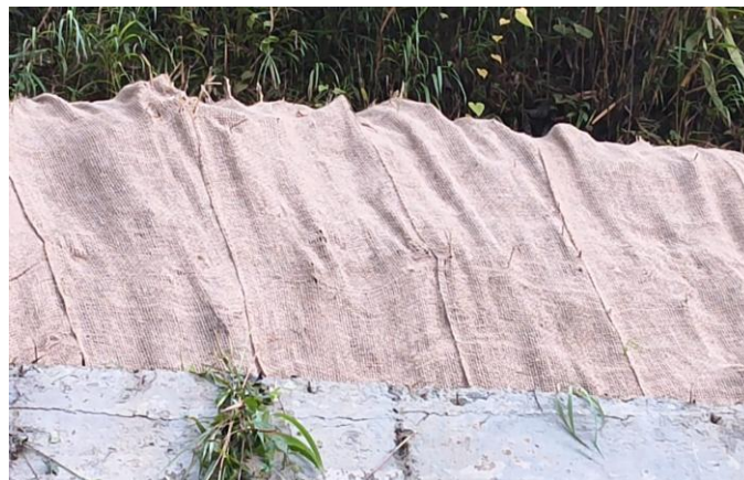
Laying of 600gsm open weave JGT
